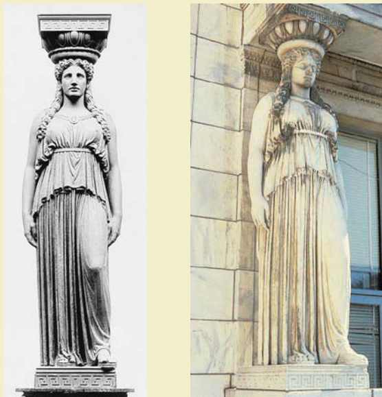
The damaging effects of acid rain can be seen by comparing these photos of a decorative statue on the Field Museum in Chicago. The first photo was taken about 1920, the second in 1990.
